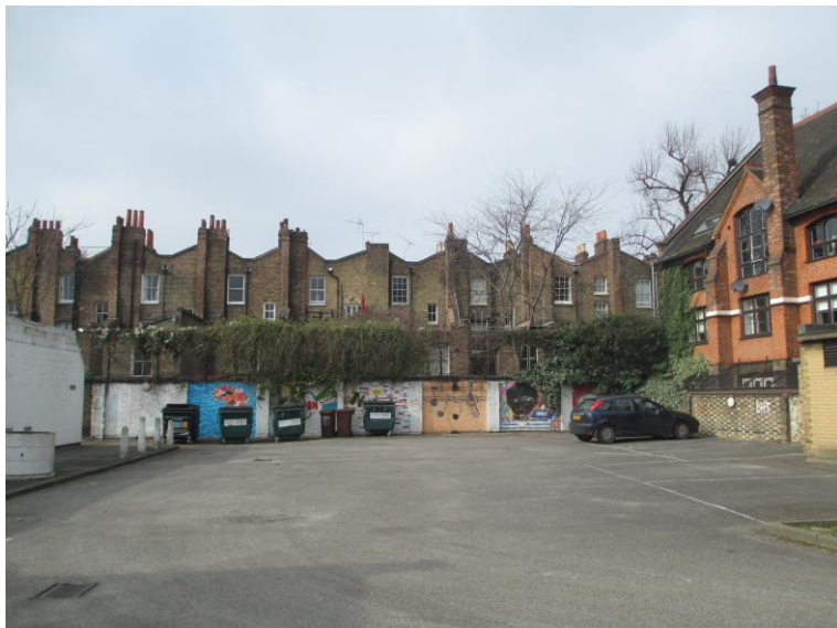
Photograph 4: The parking area and western boundary
